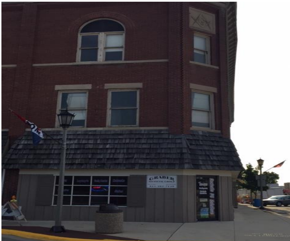
Corner of Lincoln Highway and 4 th Avenue
